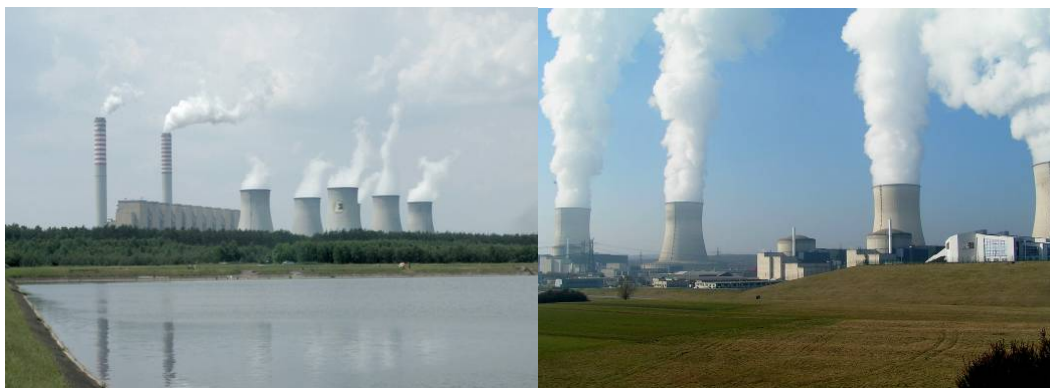
Figure 8. Coal and nuclear power plants
